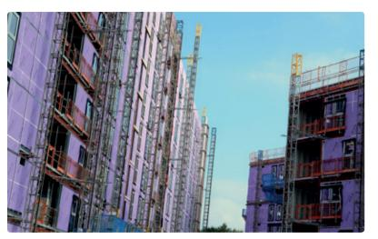
The Thrubuild® light steel framework is panelised in the factory and delivered to site for assembly. External boarding of these frames can also take place offsite depending on the system and your build process.
